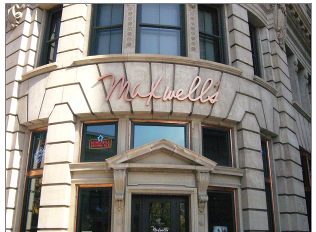
The color and material of this sign were designed to match the window cladding.
