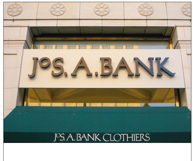
This sign on Main Street is proportional to the building and does not obscure ornamental details.
