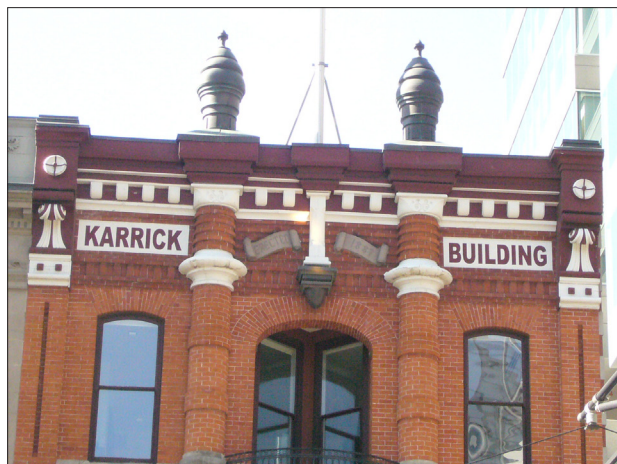
Wall signs should be relatively flush with the facade of the building.
