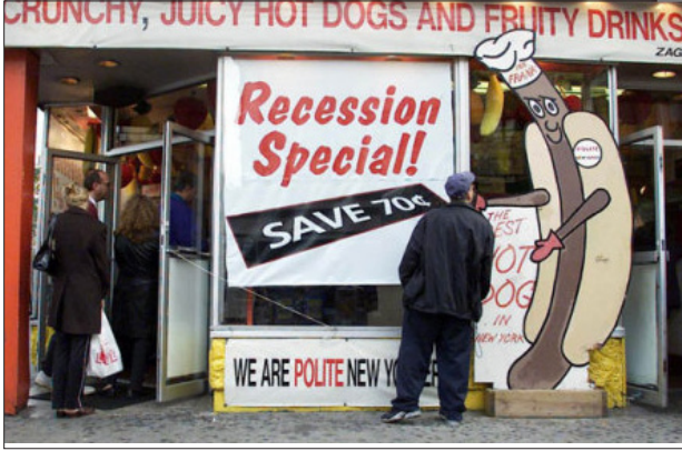
Signs that cover significant architectural details are discouraged.
